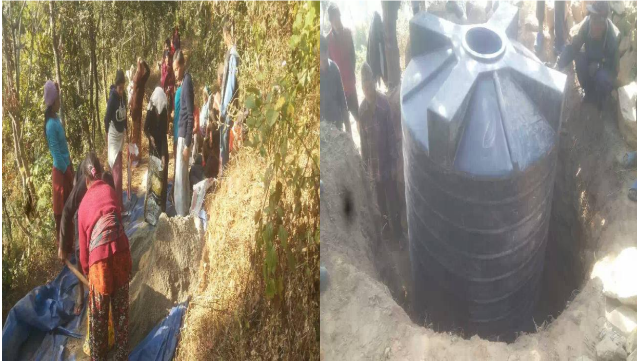
Figure 2: Participation of community members, and water tank installation
