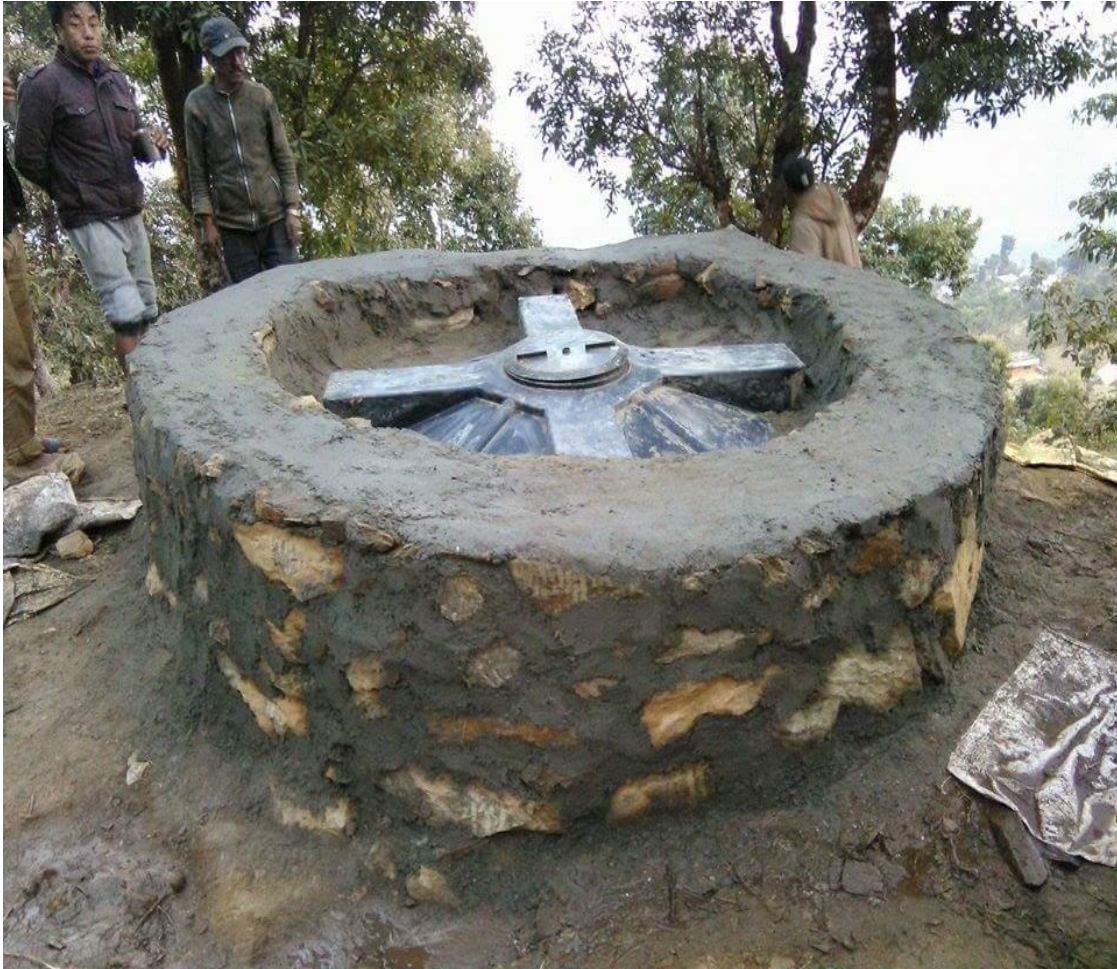
Figure 4 : 5000 liter water tanks on the reservoir R1.
