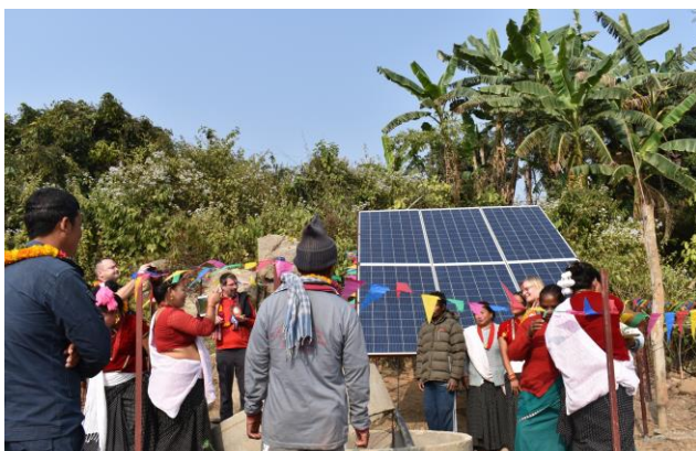
Installation of solar water pump.
