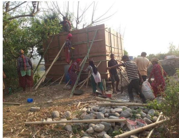
Construction of RCC water storage tank.
