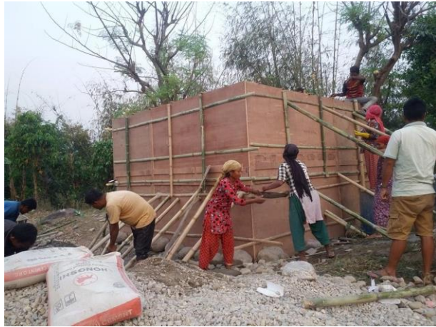
Construction of RCC water storage tank.
