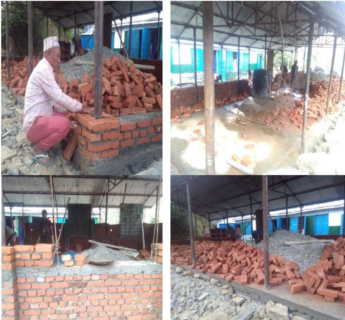
Figure: Construction work of Setidevi Primary School
