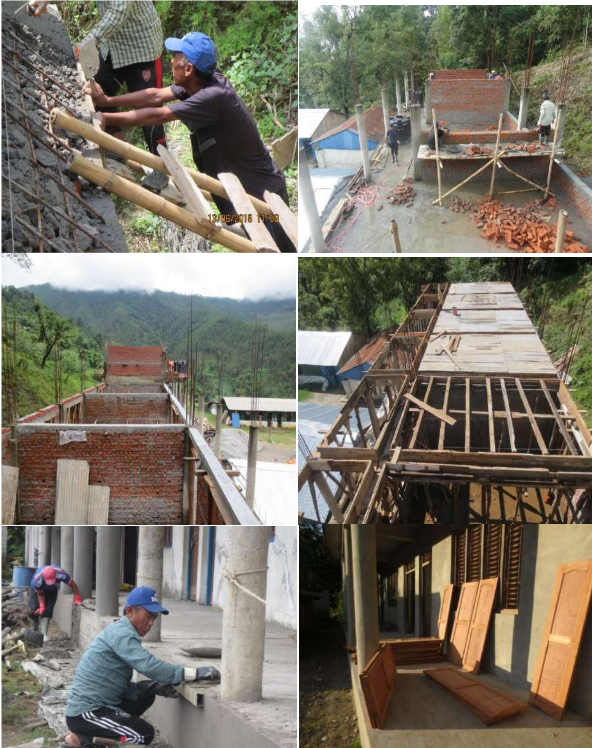
Figure: Construction work of Jalpadevi Secondary School
